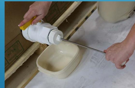
5) Once retracted, close the valve before you remove the plunger cutter. Once the cutter is removed, hook your equipment up to the 2" female NPT threads on the valve.
