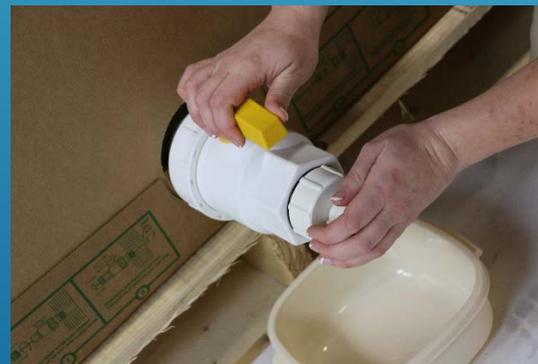
4) Place a small tray or bowl under the valve. This will be for the small amount of liquid you will lose when you remove the cutter. Retract the arrow portion.
